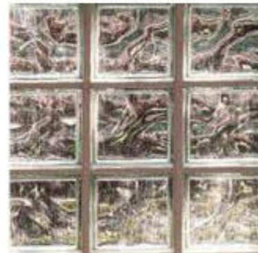
EXISTING GLASS BRICK
